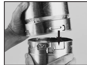
Line up the pipe ends.
