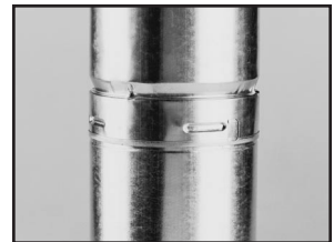
Push the ends of the pipe together.
