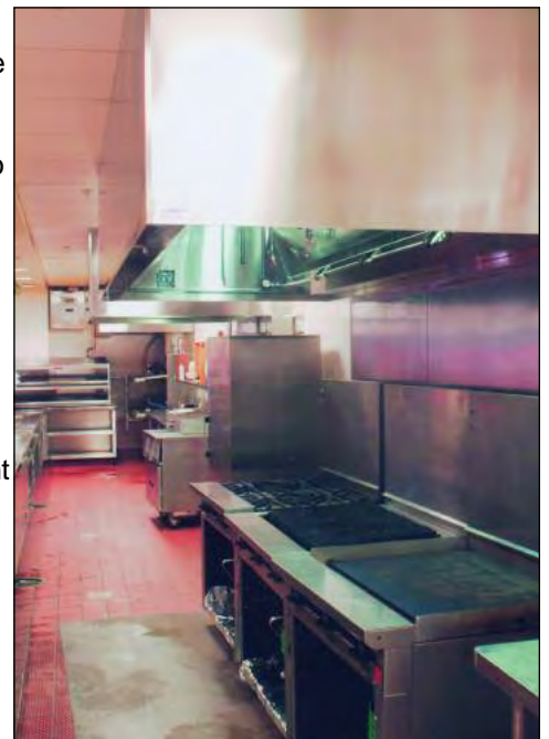
Fifteen new hoods were installed.
