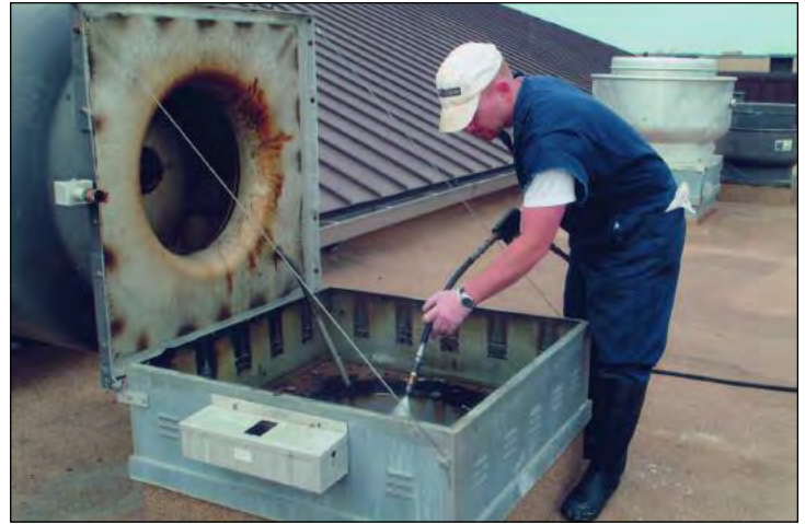
Spraying from roof down, no leaks below.
