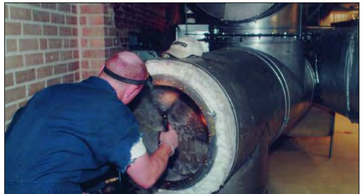
Cleaning process requires no brushing or scraping.
