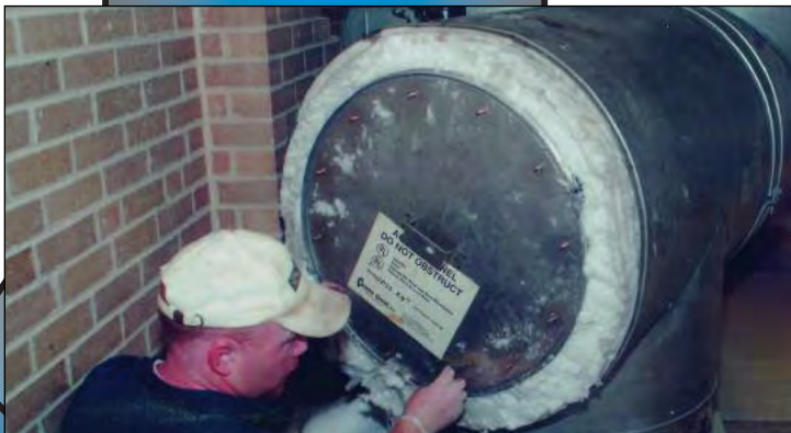
Quick access cleanout covers speed cleaning time.
