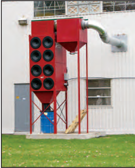
RP8 with Spark Arrestor
