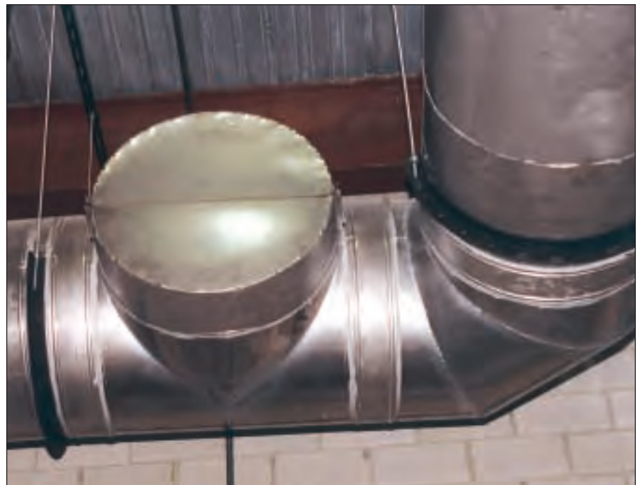
Easily accessible inspection/clean-out ports reduce service time and cost.
