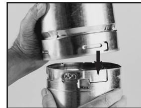
Line up the pipe ends.
